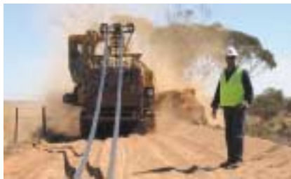
Murraylink underground cable rollout
