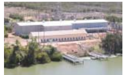
Red Cliffs Converter Station
